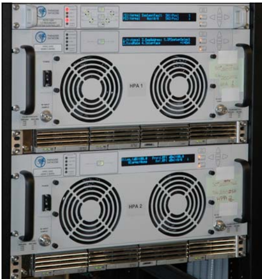
◀ 400W C-Band (4RU) 1:1 Phase Combined System
